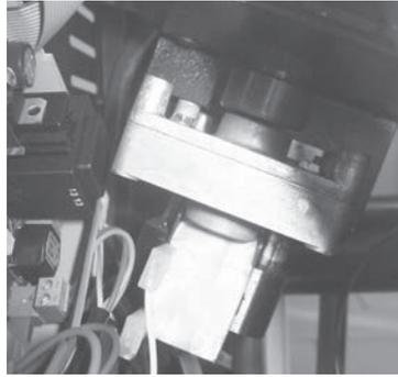
**Reduction motor:** if the motor stops, the thermostove continues to function until the flame goes out for lack of fuel, and until it has cooled down to the minimum level.
